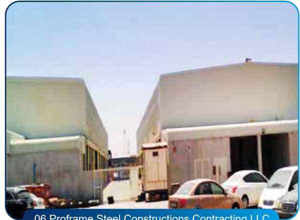
06 Proframe Steel Constructions Contracting LLC
